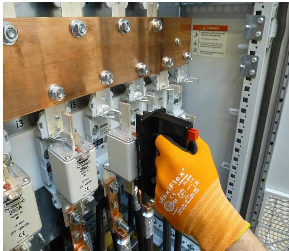
Figure 5-4 Mounting the fuse
