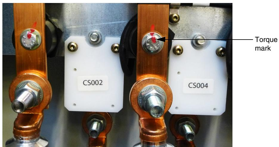
Figure 5-1 Torque marks
