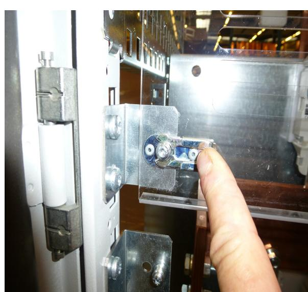
Figure 4-7 Unclipping the internal safety barriers
